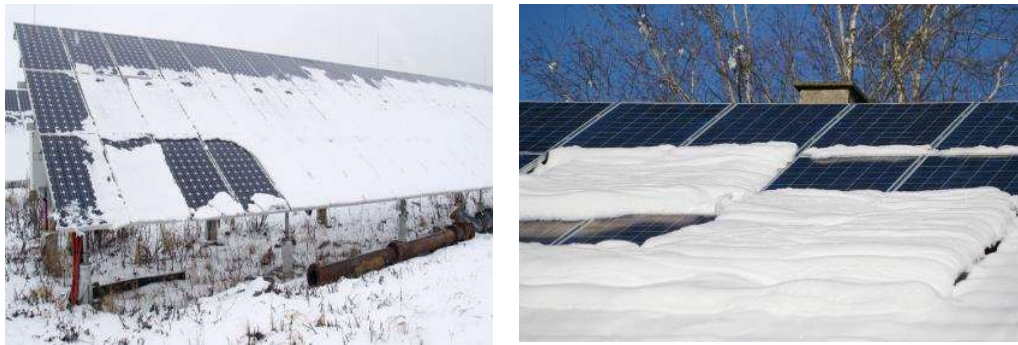
Figure 1.5 Snow accumulation on PV systems. (Ref: https://solarbuildermag.com/ )
