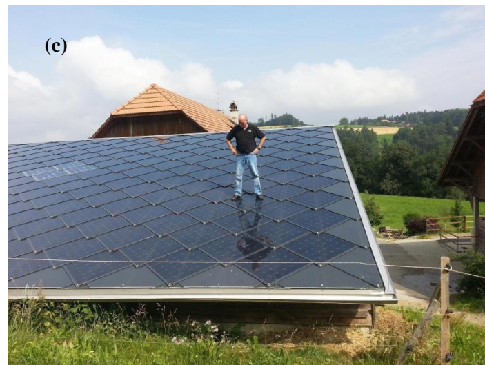
Figure 2. Different ways of PV panels arrangement such as (a) vertical, (b) horizontal and (c) diagonal [81].
