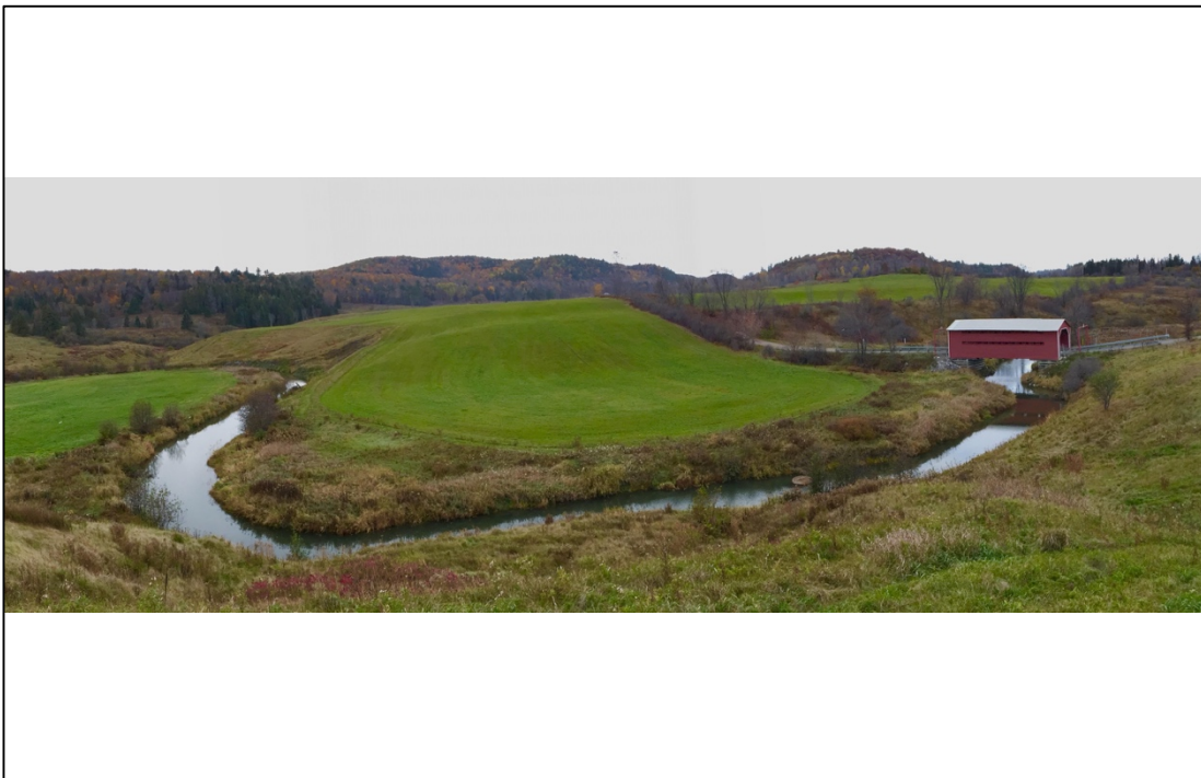
Figure 5.25 CP3 – Pont couvert
